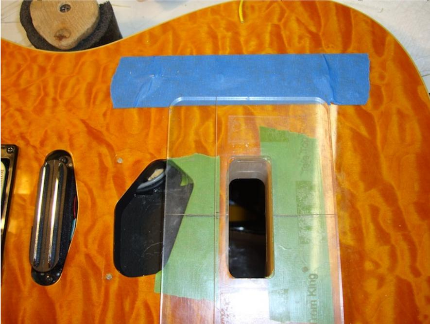
7. Remove template but leave tape with centerline and scale length. Drop TKS-2/3 unit in and make sure it centers.
